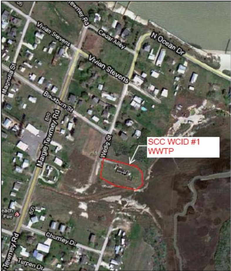
Figure 3-6 SCC WCID #1 WWTP
