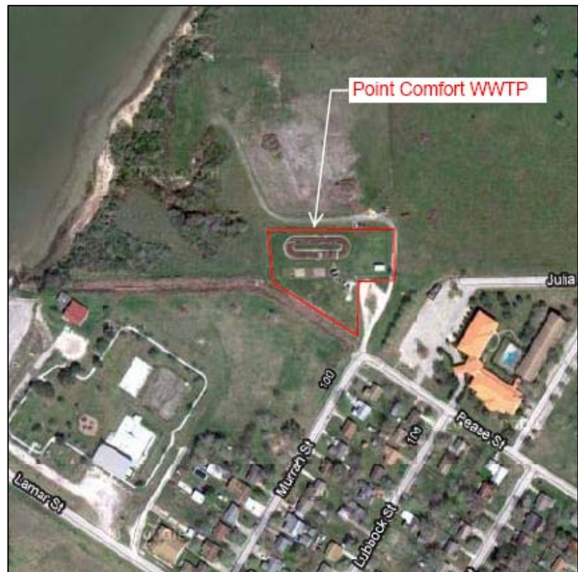
Figure 3-1 City of Point Comfort WWTP
