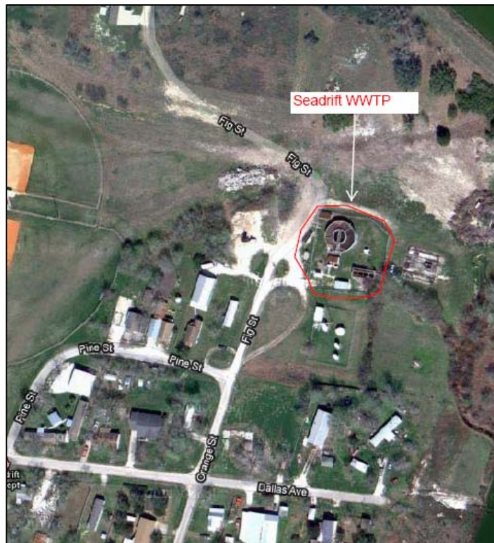
Figure 3-3 City of Seadrift WWTP
