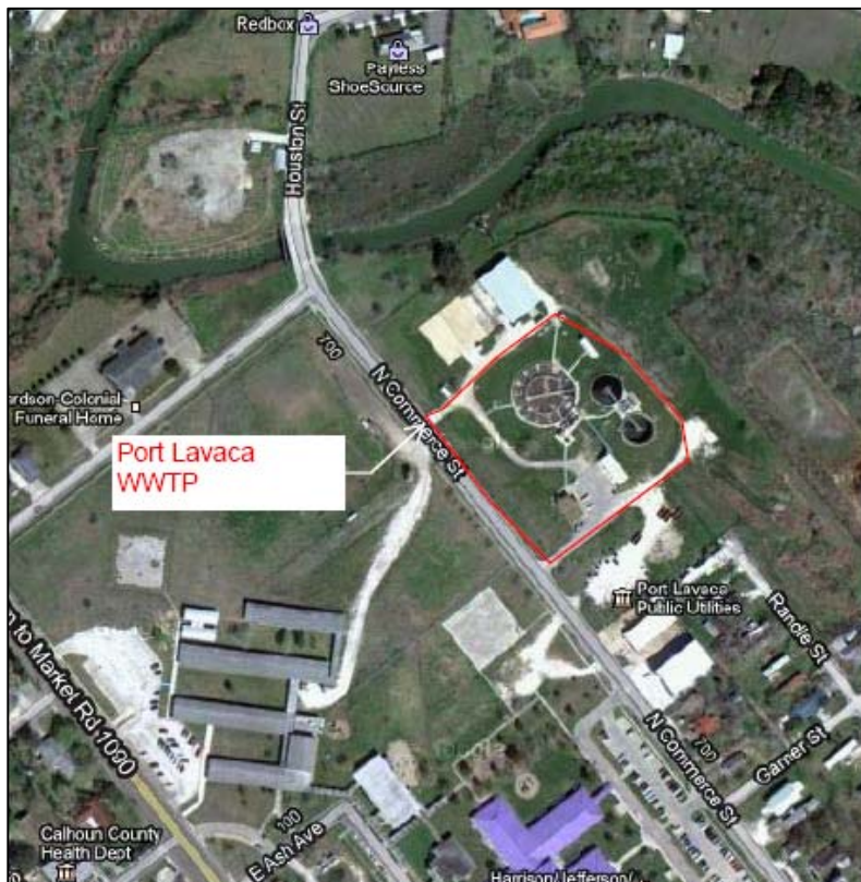
Figure 3-2 City of Port Lavaca WWTP
