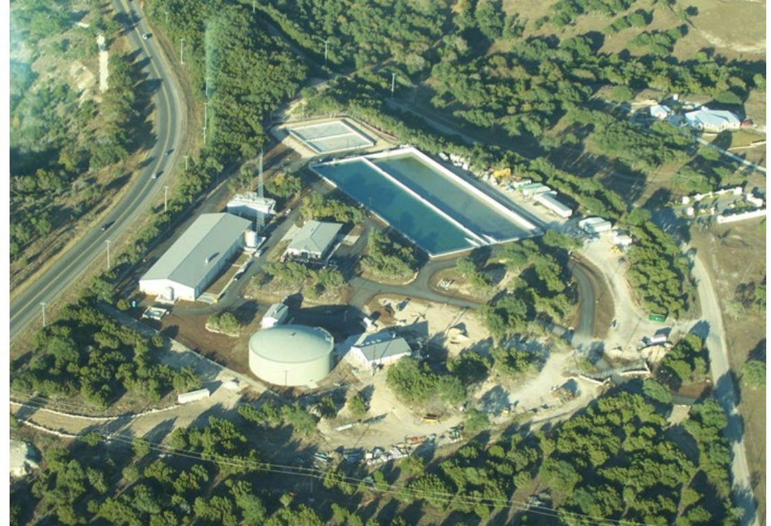
Western Canyon WTP
