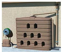
Rainwater harvesting has gained popularity as different sizes and shapes of tanks are emerging. Below ground rainwater tanks and smaller cisterns are available to offset municipal water use. The water from the cisterns can be for potable and non-potable use.
