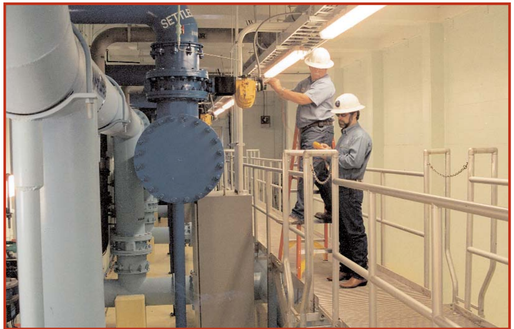
Plant Operators Dan Drugan and Garry McAlpin calibrate a filter valve in the filter gallery beneath the San Marcos Regional Water Treatment Plant
