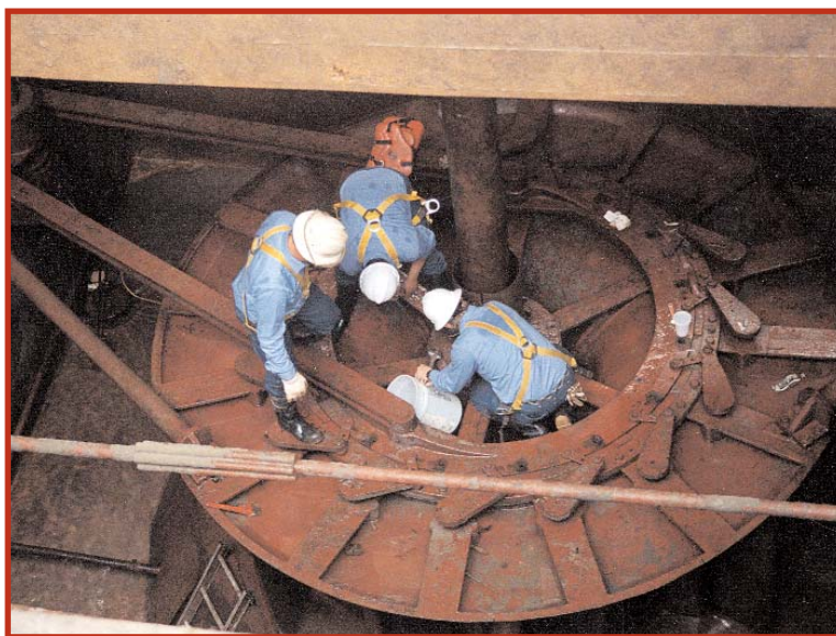
Deep inside a hydroelectric powerhouse, crew members conduct a turbine inspection in preparation to adjusting the bearing blocks.
