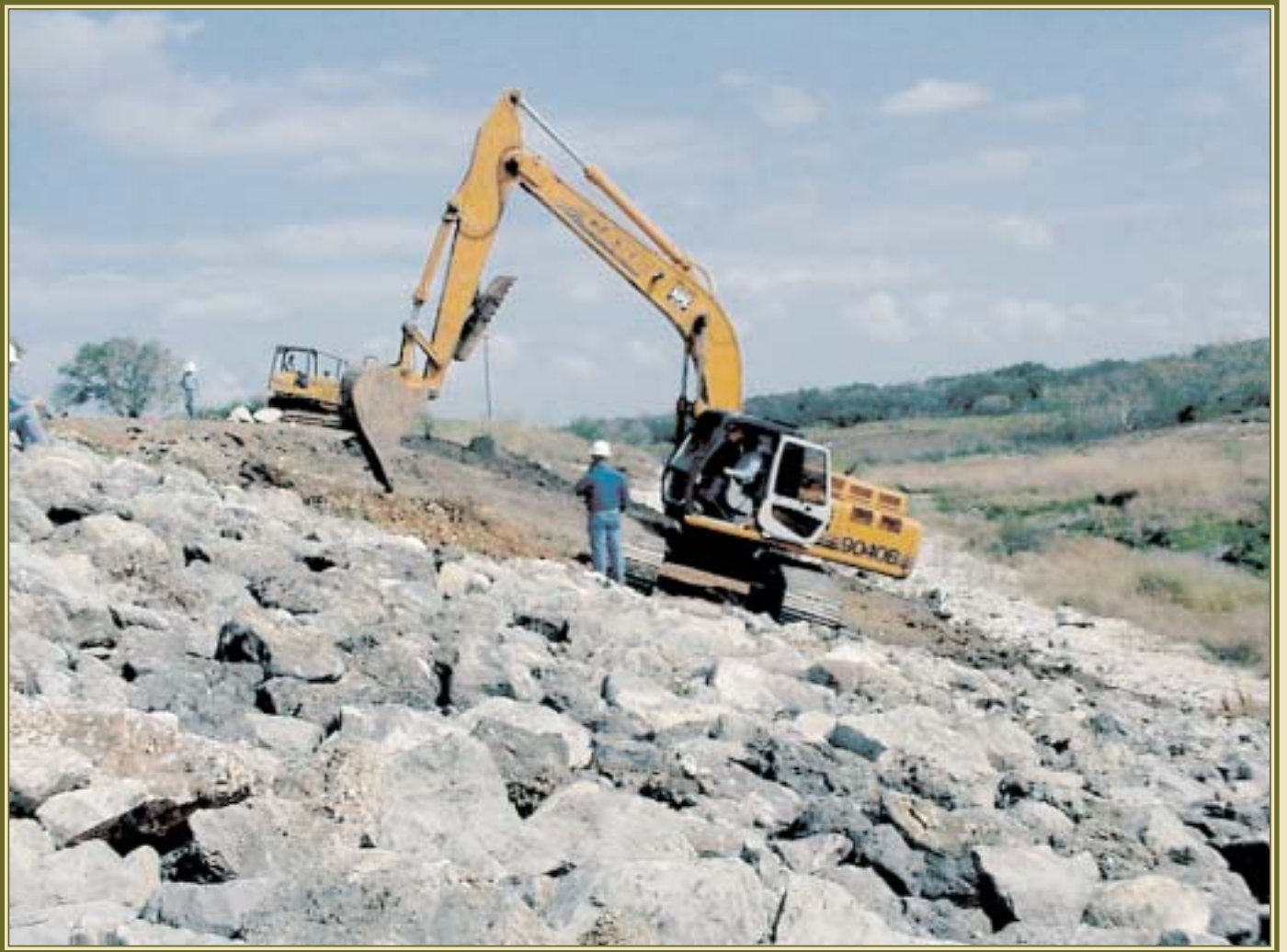
As part of a major erosion control project, GBRA employees place the last of 900 tons of rip-rap on the north slope of the Coletto Reservoir main spillway discharge channel.
