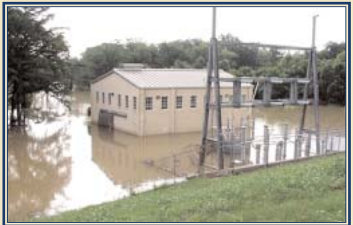
GBRA's Canyon Hydroelectric Plant will be out of operation until Summer 2003 to repair approximately $1.8 million of flood damage.
