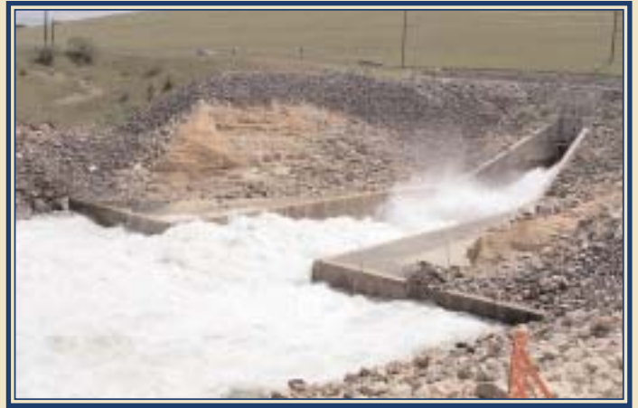
Floodwater from Canyon Reservoir churns through the release gate at the base of Canyon Dam at rates up to 5,000 cfs.
