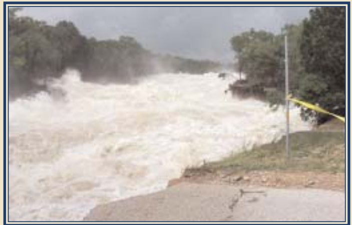
Floodwater pouring down the spillway channel completely cuts through the access road to Canyon Dam.
