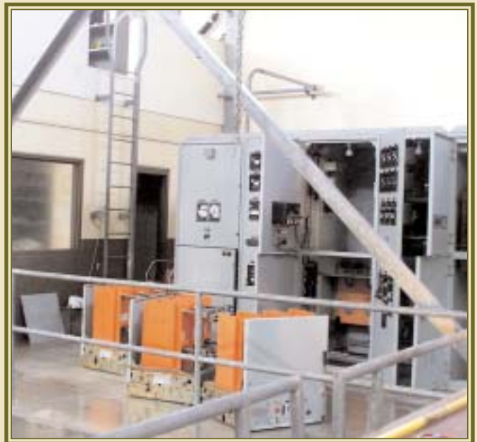
Eleven feet of floodwater damaged a majority of the switchgear at the GBRA Canyon Hydroelectric Plant.
