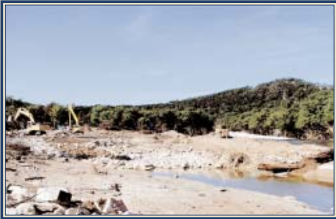
Contractors begin the immense task of removing tons of rock washed into the Guadalupe River channel from the emergency spillway.
