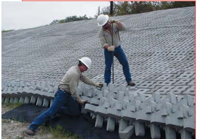
GBRA Coleta Creek employees install concrete revetment mats as part of an erosion repair project on the Main Dam spillway discharge channel.
