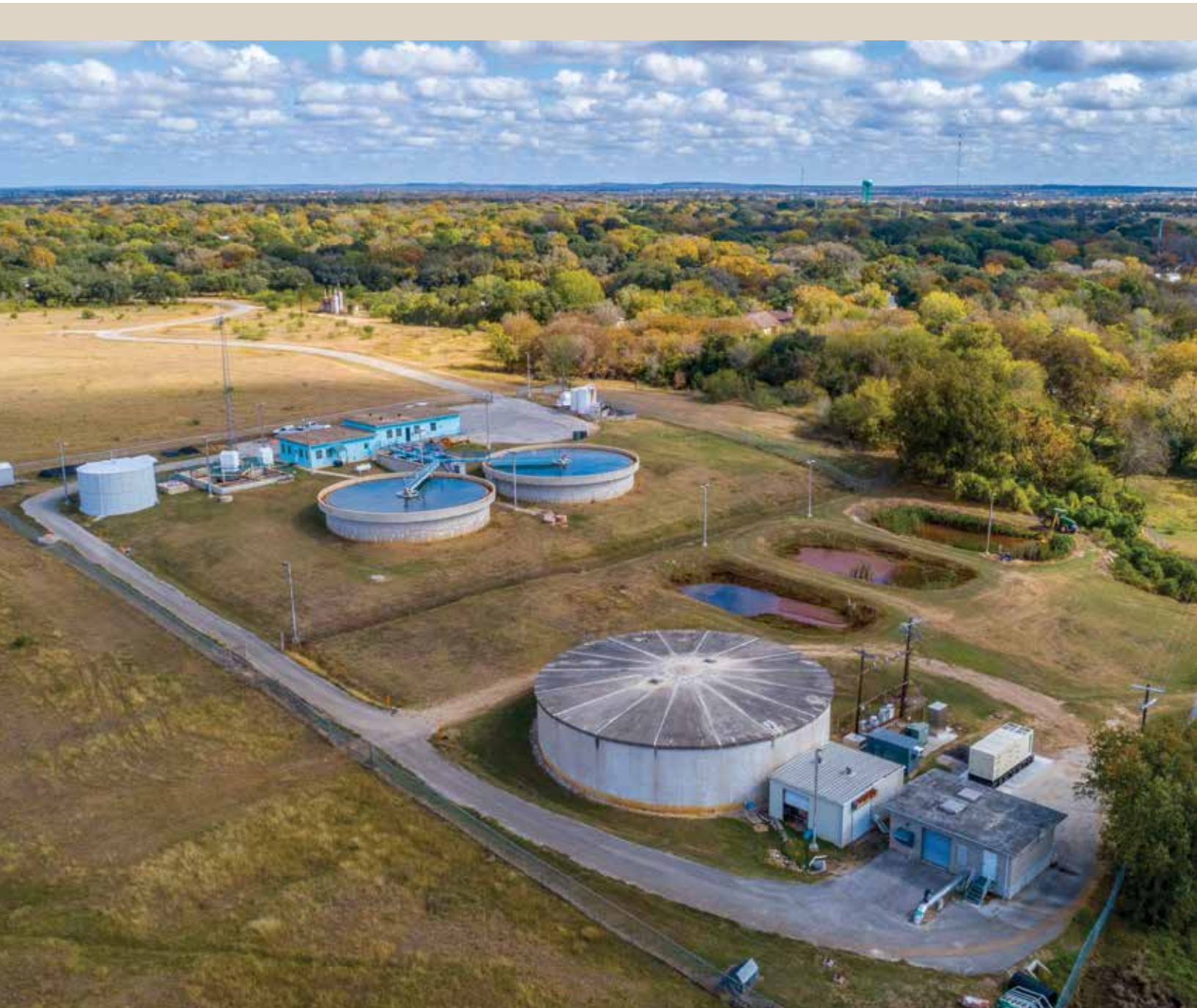
Aerial view of the Luling Water Treatment Plant. Surface water from the San Marcos River is treated here and delivered to the cities of Luling and Lockhart for distribution. The plant was constructed in 1978 and has a treatment capacity of 2.5 million gallons per day (MGD).
