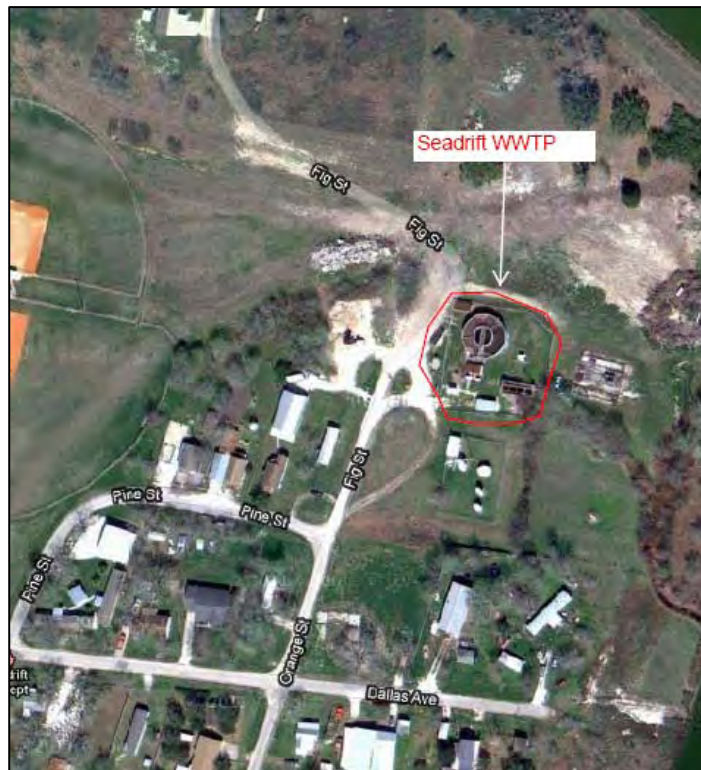
Figure 3-3 City of Seadrift WWTP
