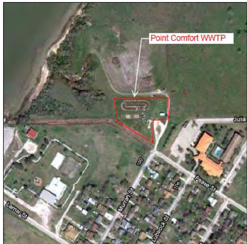
Figure 3-1 City of Point Comfort WWTP
