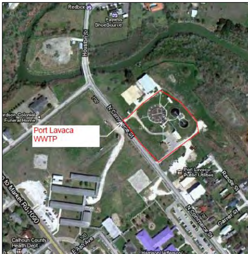
Figure 3-2 City of Port Lavaca WWTP
