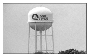
The George St. water tower rehabilitation began in December of 2002, and was complete ed in April of 2003. The project consisted of sandblasting and repainting the exterior of the structure and also the sandblasting, painting, and coating of the interior bowl surface. In addition, the City logo was added on the east and west sides of the bowl.
