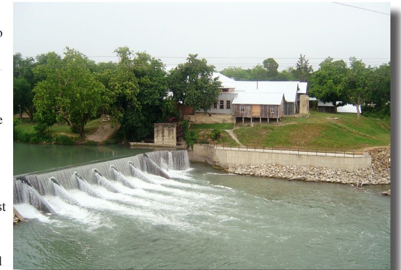
The City of Luling receives most of its water from the San Marcos River, shown here at the old Zedler Mill and Dam in Luling.
