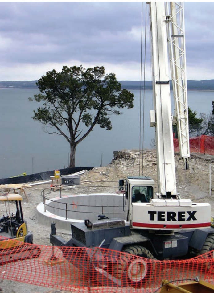
Construction of a raw water intake wet well at Western Canyon Water Treatment Plant. A hole, 18 feet in diameter, was bored 140 feet into limestone to draw water from Canyon Lake.
