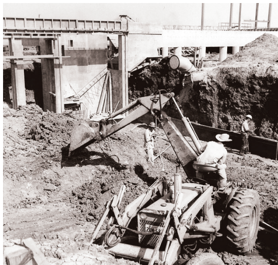
LEFT - Excavation to place underground piping during the construction of the Port Lavaca Water Treatment Plant, September 22, 1969.
