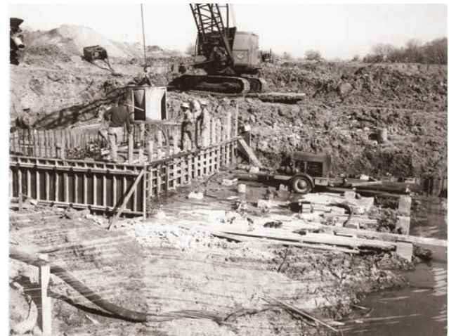
BELOW – Pouring the foundation slab for the Saltwater Barrier and Diversion Dam on the Guadalupe River at the confluence with the San Antonio River in Calhoun County, February 26, 1965.
