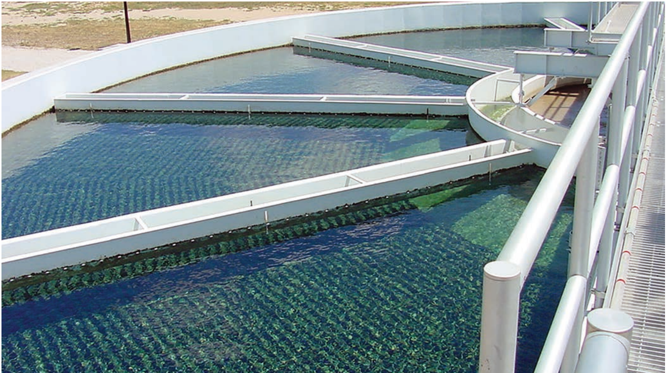
Clarifiers at the San Marcos Water Treatment Plant are used in the water treatment process to settle coagulant and dirt in raw river water. The clear water then travels through troughs to the filtration and disinfection process before being pumped to the city of San Marcos.
