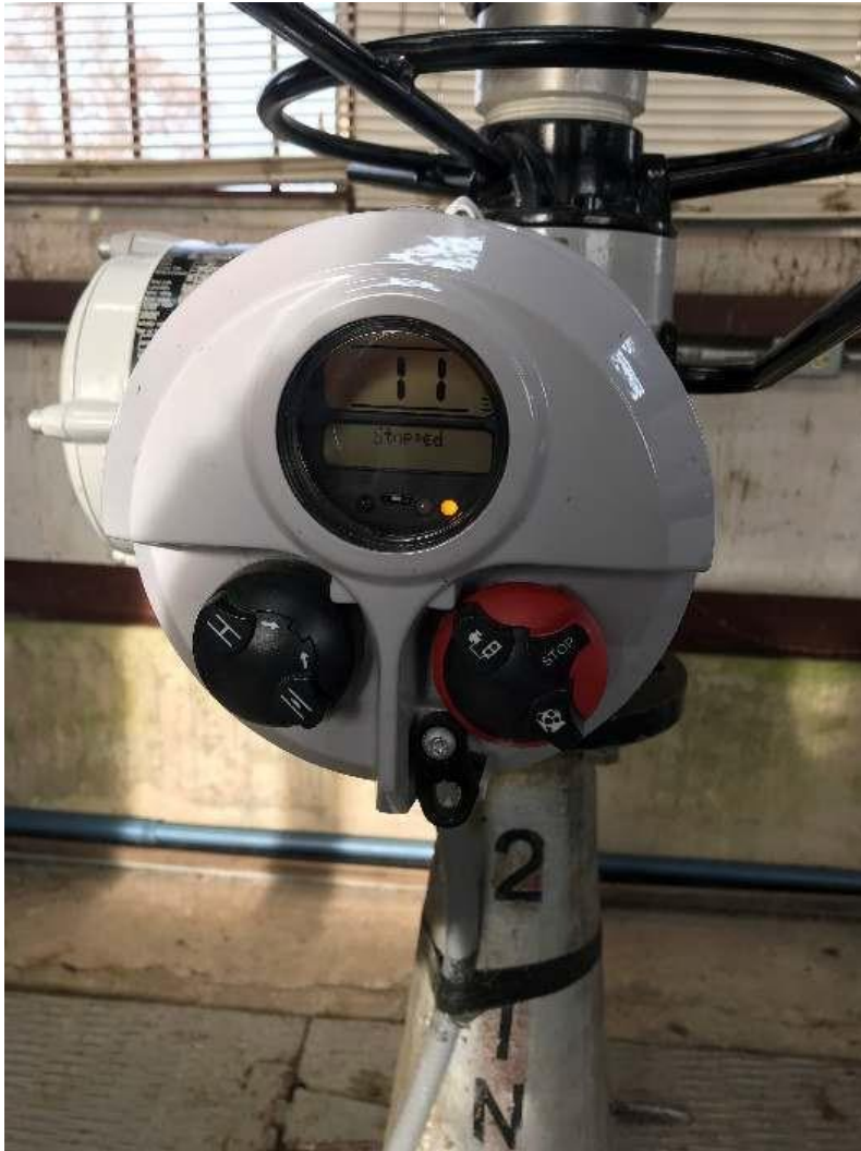
Figure 31. Detail of TP-1 electronic spillgate control actuator for bay 2 intake, ca. 2000, looking southwest
