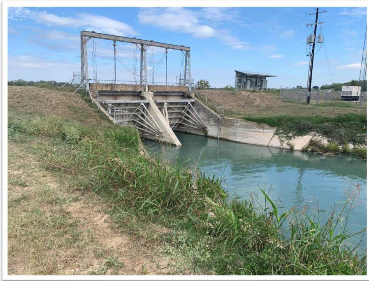
Figure 38. TP-1 Tainter headgates with lifting frame, October 2020, looking north
