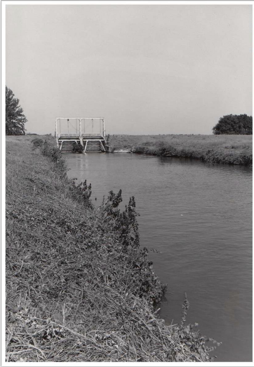
Figure 28. TP-1 by-pass canal with control gates and lifting frame at TP-1 emergency spillway, ca. 1965, looking north
