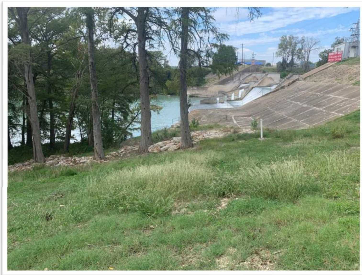
Figure 36. TP-1 north embankment with downstream armoring and fishway pier, October 2020, looking west
