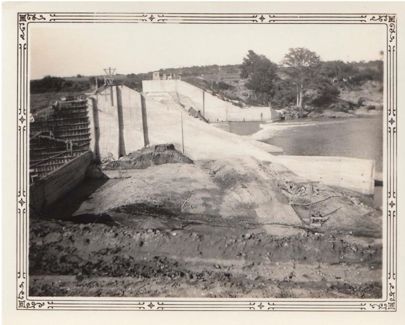
Figure 24. TP-1 right (south) embankment and retaining wall under repair with north regulating pier and control house (background), ca. 1932, looking east
