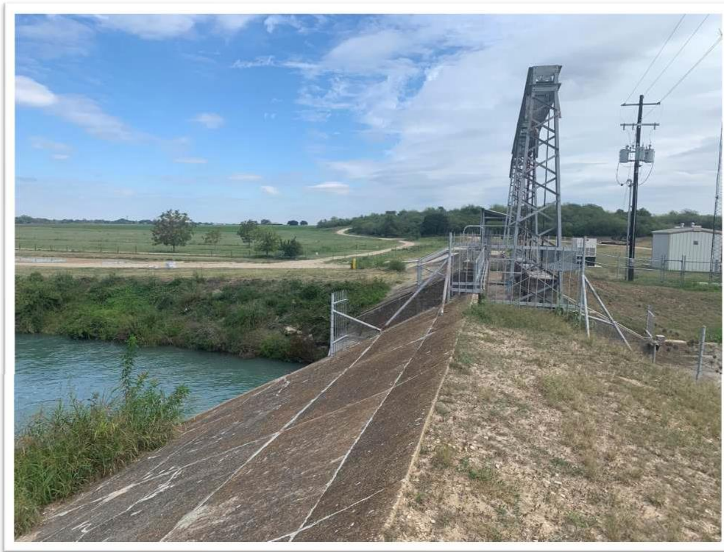
Figure 37. TP-1 diversion canal and headgate lifting frame, October 2020, looking northeast
