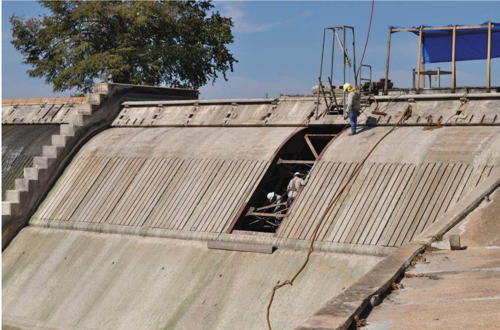
Figure 29. Replacement of TP-1 spillgate timber facings, ca. 1980, looking northwest
