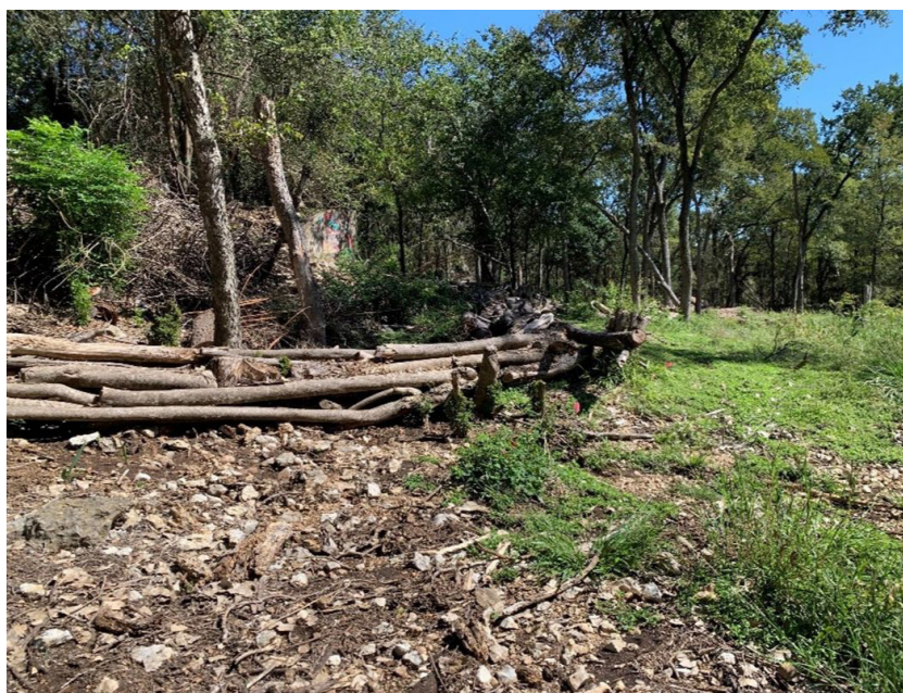
Completed Vegetative Filter Strip in Sessom Creek Natural Area
