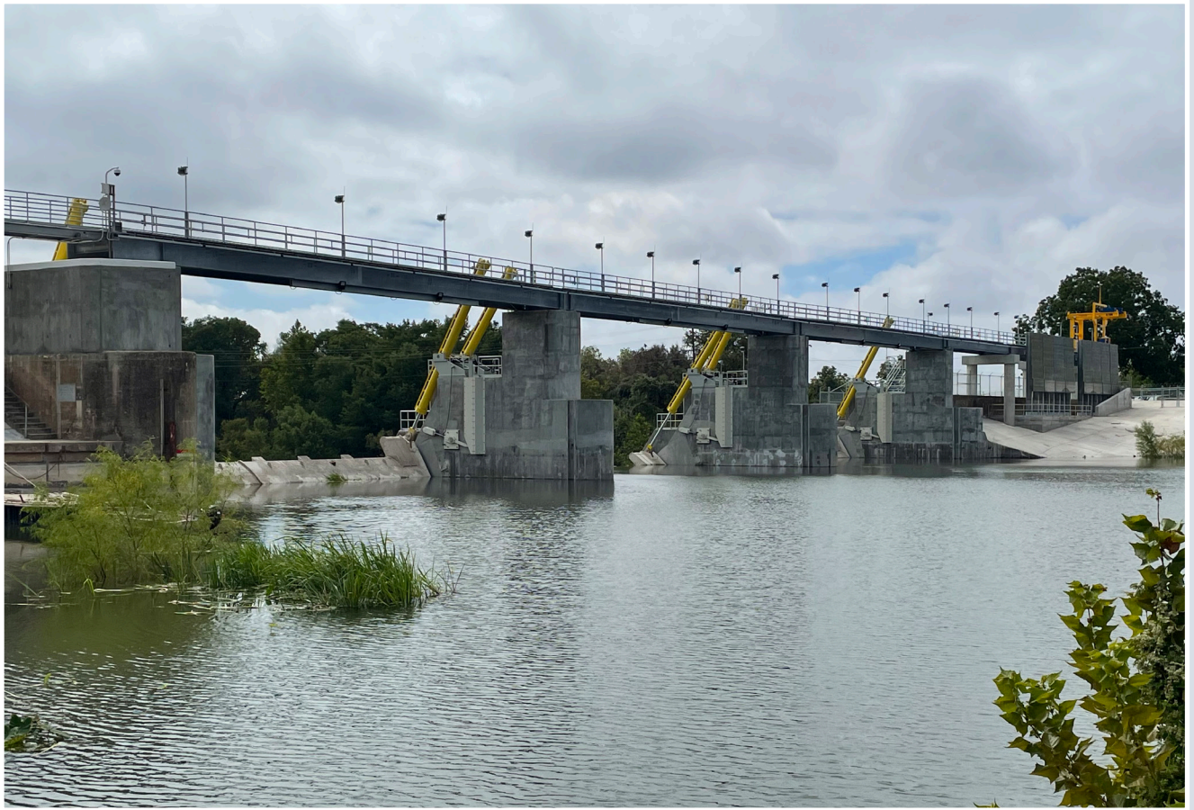
Rehabilitation of the hydroelectric dam at Lake Dunlap is nearing completion
