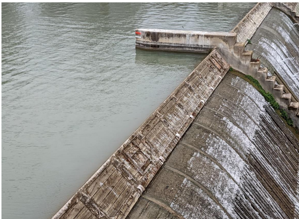
N. Lake McQueeney Dam (TP-3) showing close-up of wood used in bear trap gates. View North. File: PXL 20220308 165624889
