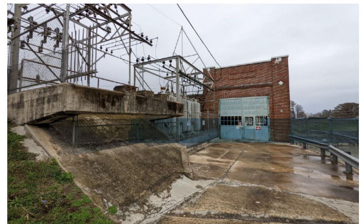
Lake McQueeney Dam powerhouse.
