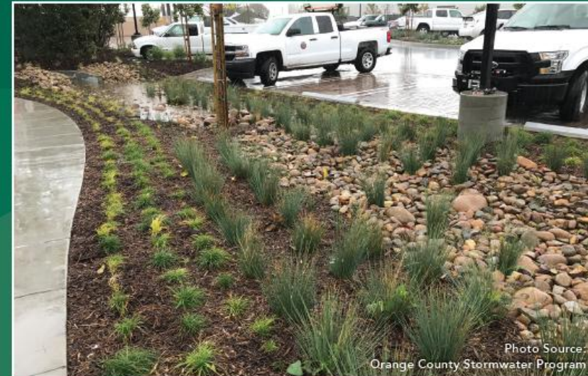
Bioretention area next to permeable parking spaces.
