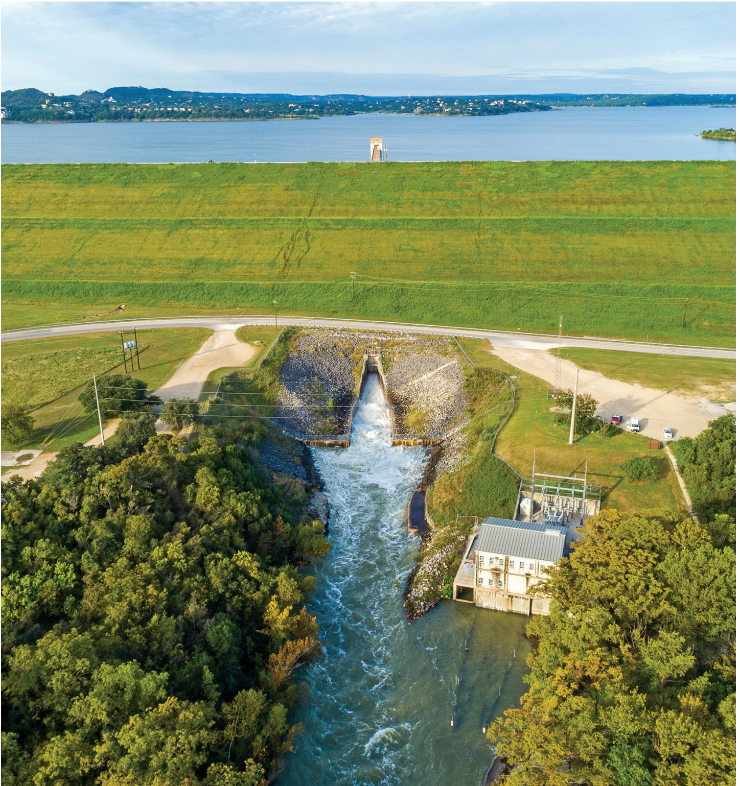
View of Canyon Lake Reservoir/Dam and Canyon Hydroelectric Plant
