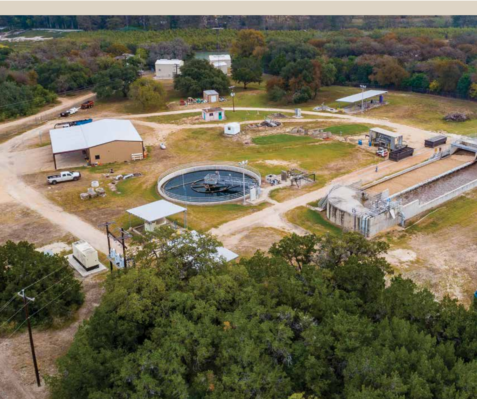
Stein Falls Water Reclamation Treatment Plant servicing the FM 725 area south of New Braunfels was expanded in 1985, 1996 and 2006, and is currently permitted to treat 0.95 MGD.
