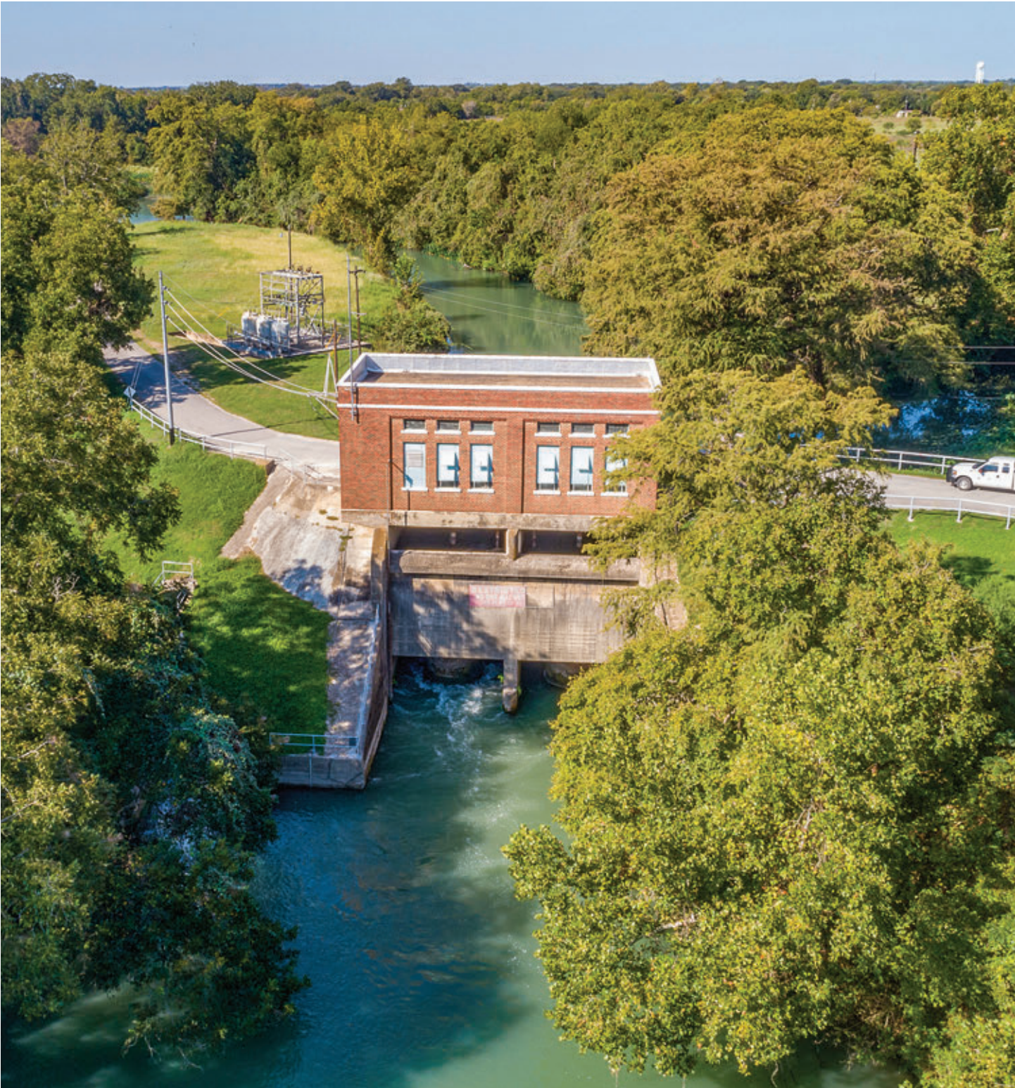
Built in 1927, the Nolte Hydroelectric Plant is about 2.5 miles (channel distance) below TP-5 Dam (Lake Nolte) on the Guadalupe River, and 3 miles southeast of Seguin, Guadalupe County.
