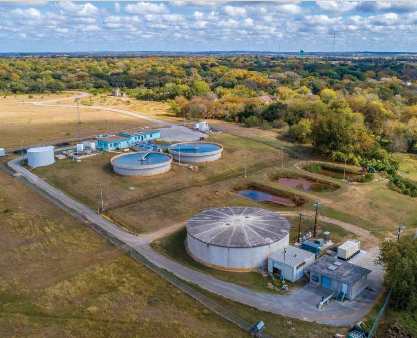
Aerial view of the Luling Water Treatment Plant. Surface water from the San Marcos River is treated here and delivered to the cities of Luling and Lockhart for distribution. The plant was constructed in 1978 and has a treatment capacity of 2.5 million gallons per day (MGD).
