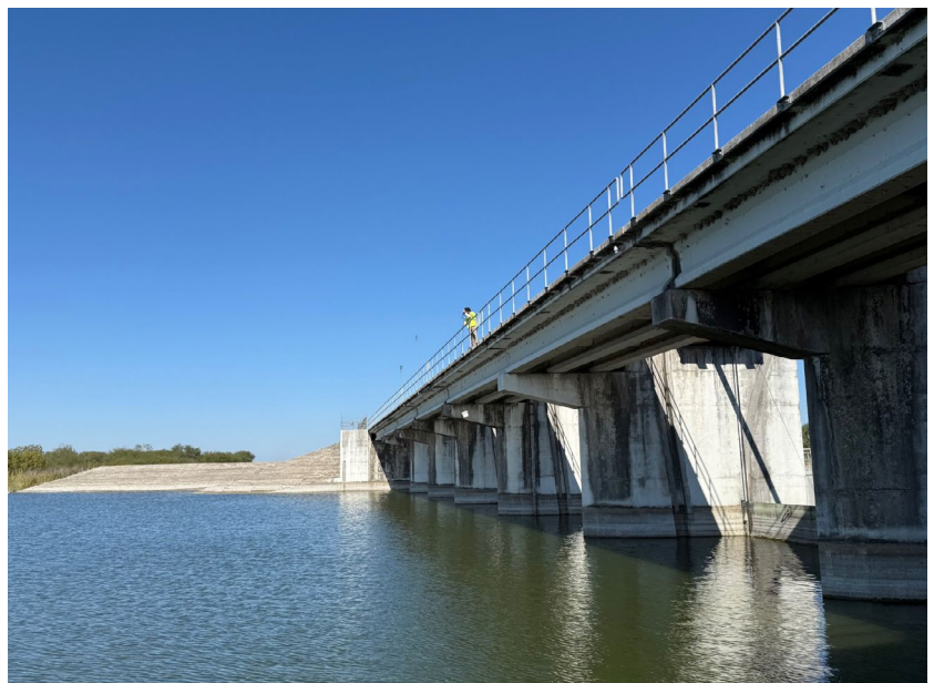
Sampling at Coledo Creek Dam.
